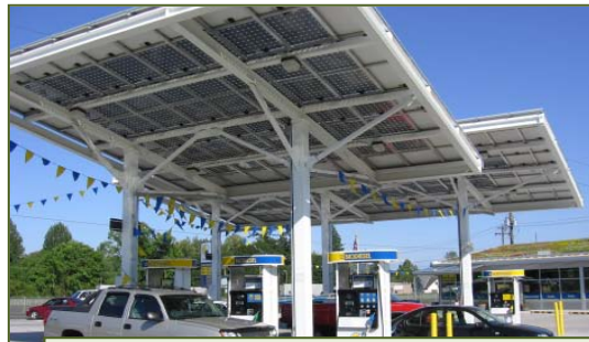
Sustainable redevelopment of a remediated brownfield site formerly used as a gasoline station in Eugene, OR, focused on building a biofuel station with solar power along with low impact development elements such as bioswales; the biofuel is made of discarded cooking oil collected across the state.
