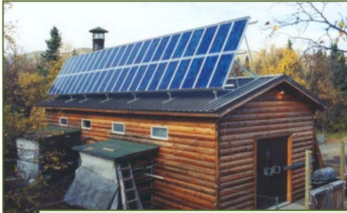
An off-grid PV system at Brooks Camp, AK, powered an air sparging pump that operated only during daylight hours, which sufficiently treated contaminated groundwater while avoiding energy loss and freeze potential associated with battery storage.
