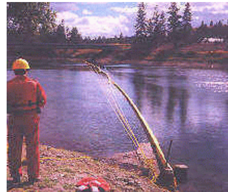
Figure 3-2: Boom deployed across Big Bear Creek.
